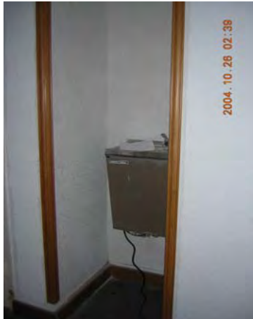
Electric water cooler in corridor recess in violation of current accessibility requirements.
