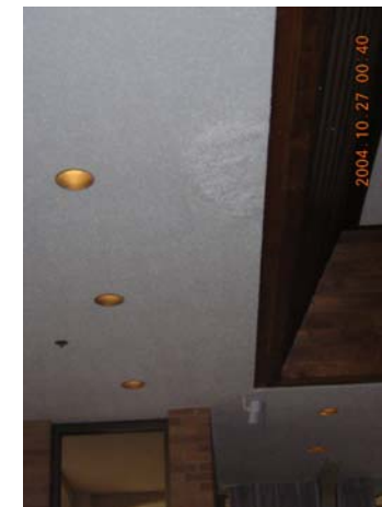
Water damage observed in ceiling of ground floor lobby.
