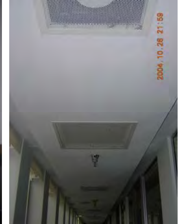
Air grills and sprinkler heads in typical corridor.
