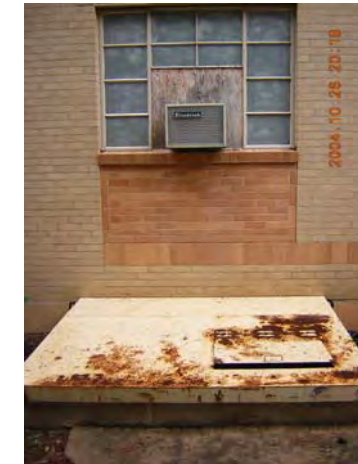
Access hatch to crawl space under the building.
