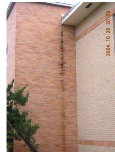
Staining from water pouring off the roof. Note the lack of control joints and cracking.
