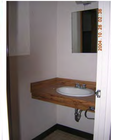
Typical lavatory and mirror in the rooms. No provisions are in place for accessibility, such as counter height or protection from drainpipes.
