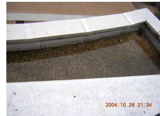
Ponding of water on lower high-rise roof.
