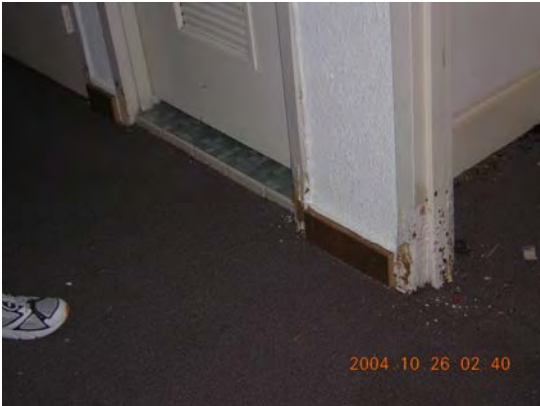
Corrosion of door jambs near toilet/shower.
