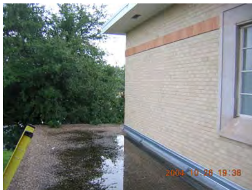
Ponding on porch roof after overnight rain.
