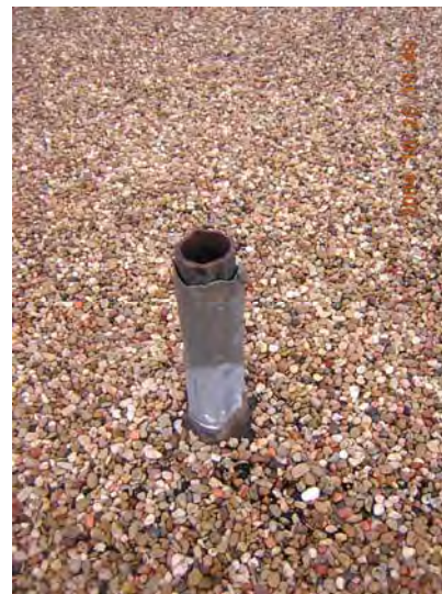
Typical roof pipe penetration with lead counterflashing in need of replacement
