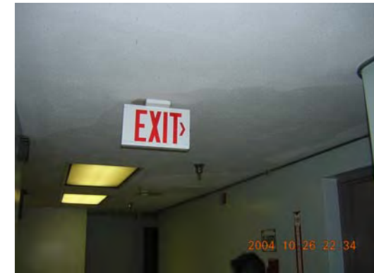
Water leak, probably from sprinkler system in the basement area laundry.
