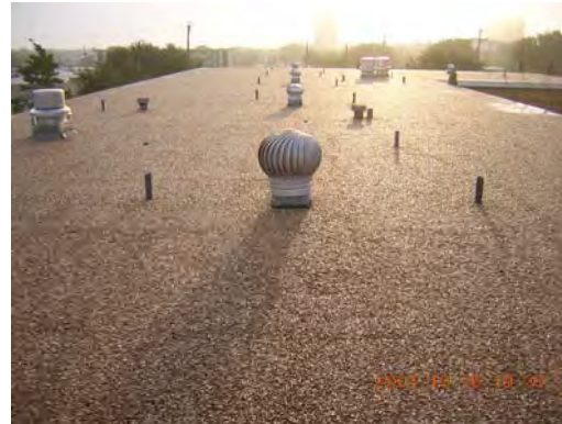
Roof on Runnels Hall looking east. Note minor ponding at the edge.
