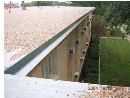
Recently installed galvanized flashing.
