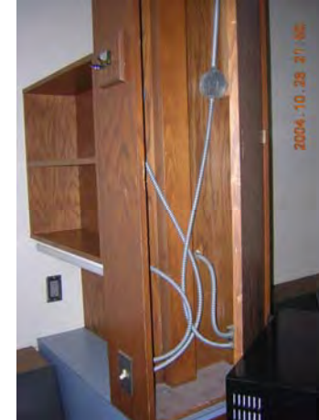
Small storage area in typical dorm room now utilized for electrical wiring.
