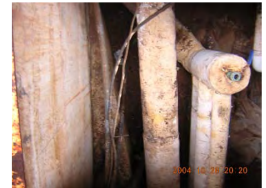
Asbestos insulated pipes in building crawl space.
