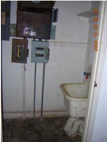
First floor utility closet containing hazardous combination of electrical boxes and janitor's sink.
