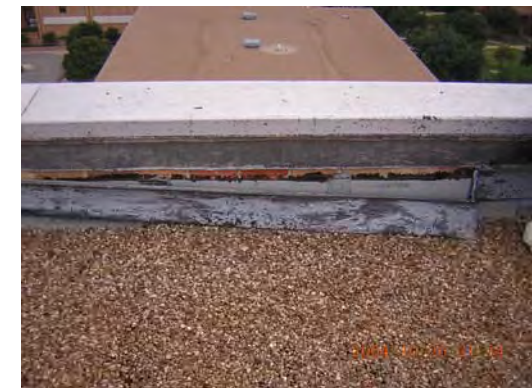
Damaged flashing on roof parapet.
