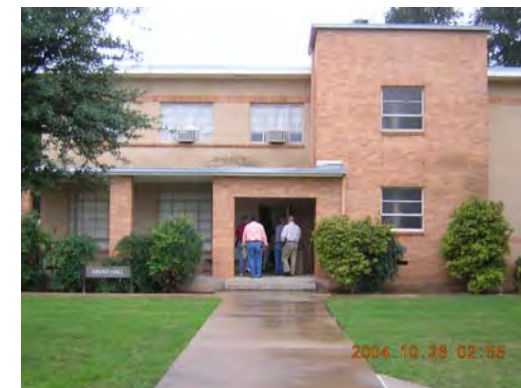
Staining from water pouring off the roof. Note the lack of control joints and cracking.
