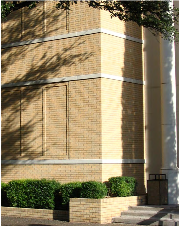
Brick with cast stone accents at the Hardeman Building
