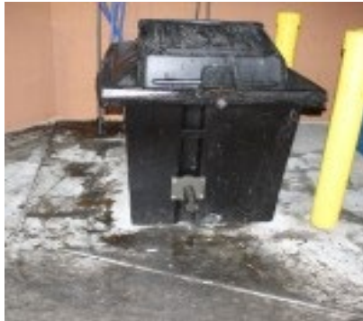
Grease leaks
